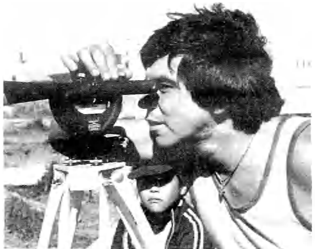
LOOKING AHEAD — Pleasant Point construction supervisor Melvin Francis, Passamaquoddy, adjusts a transit on site of planned tribal health and social services building. He expects to have a small assistant standing by. Footings are in for foundations on the one story wood frame clinic, which will measure 129 by 44 feet, plus 20 by 29 feet of office space. Work started last month; expected completion date is March 1980.
