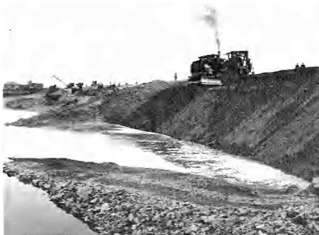
Dumping fill on Pleasant Point dam, April 1, 1936.
